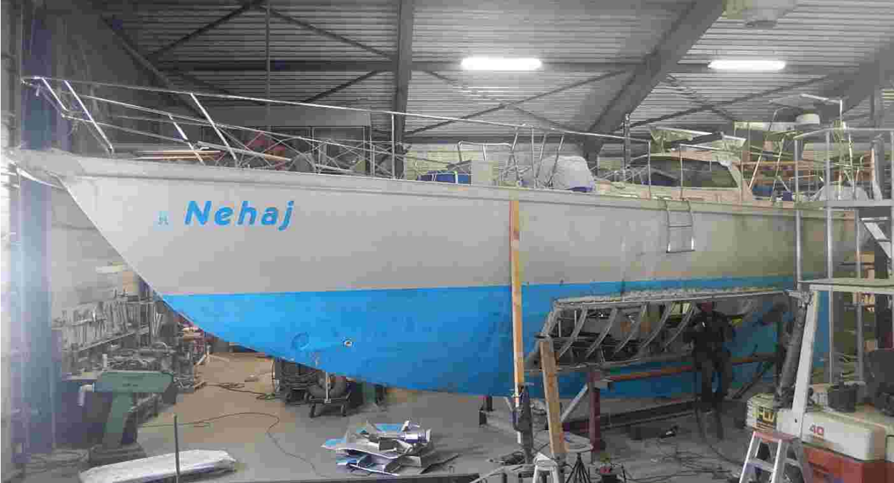
The huge area of the repair below the water line is obvious
